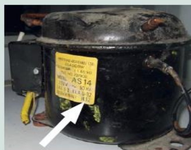
Fridge compressor marked with R12
