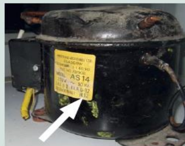
Fridge compressor marked with R12
