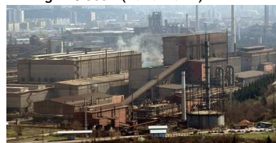
BOF STEEL PLANT Capacity : 1.068.000 t/y Design: USSR (1976)
