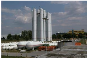
Vertical LPG Storage Vessels (250m 3 )
