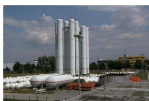
Vertical LPG Storage Vessels (250m³)
