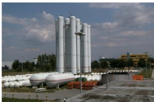
Vertical LPG Storage Vessels (250m³)
