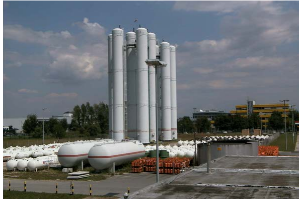
Vertical LPG Storage Vessels (250m 3 )
