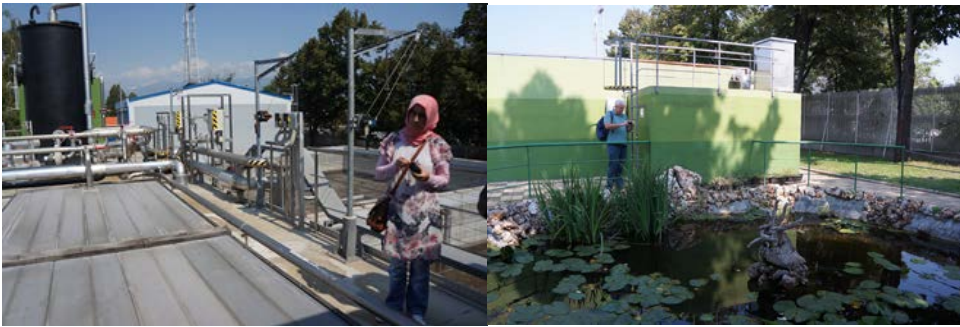
Figure 2. The treatment plant and effluent pond
