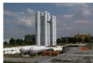
Vertical LPG Storage Vessels (250m³)
